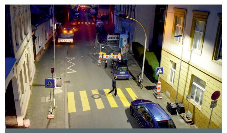
Mobile LED lighting for protecting pedestrians at zebra crossings at road works and changed road layouts.
